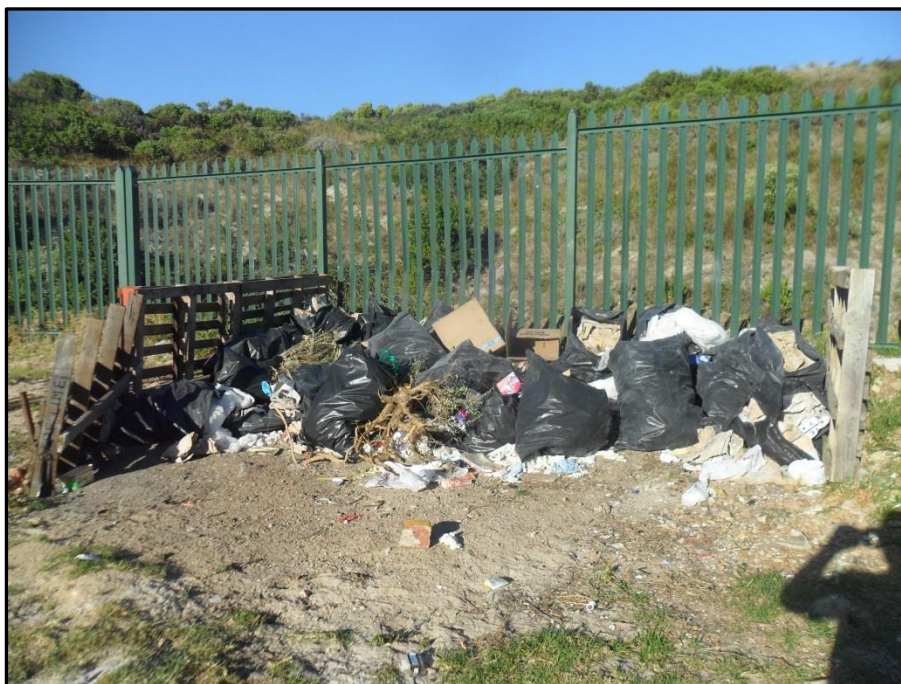
Figure 5: Waste dumped at the back of the Water Works building at Lewis Gay Dam
